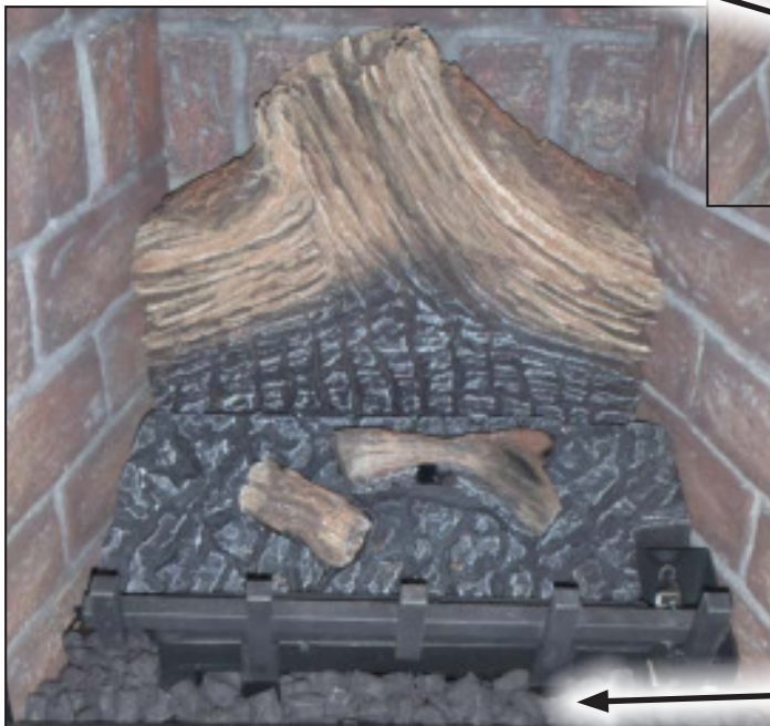
Figure 37. Coal Nuggets Installation.
