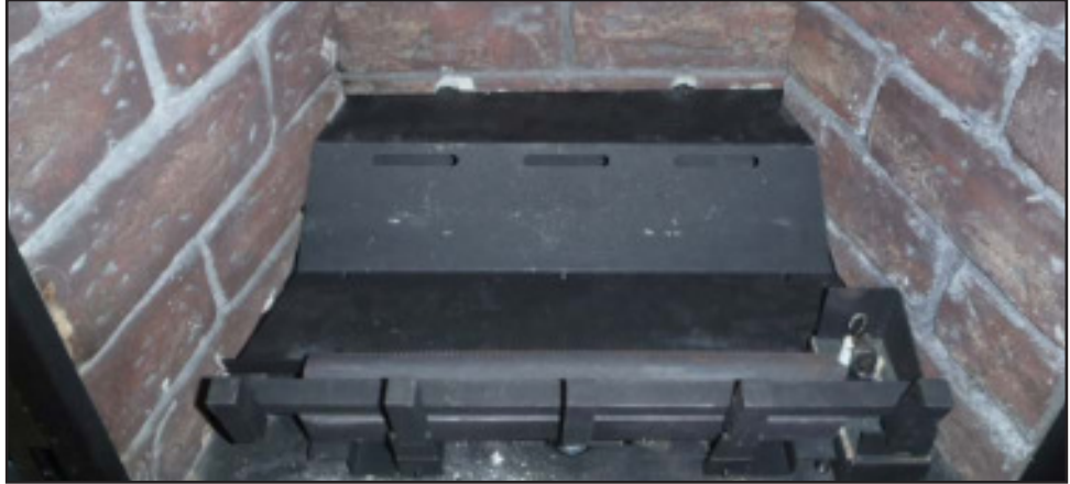
Figure 35. Empty firebox with grate and locator pins.
