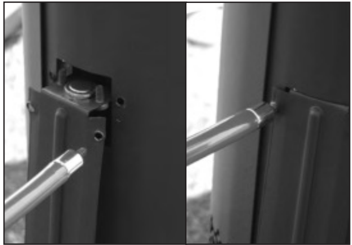
Figure 35: Spill switch installation.
