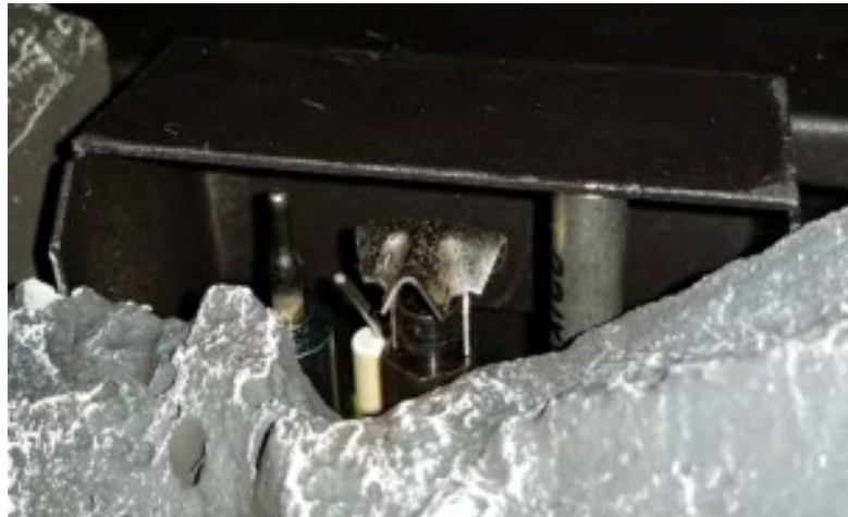
Figure 18. Pilot assembly beside the burner.
