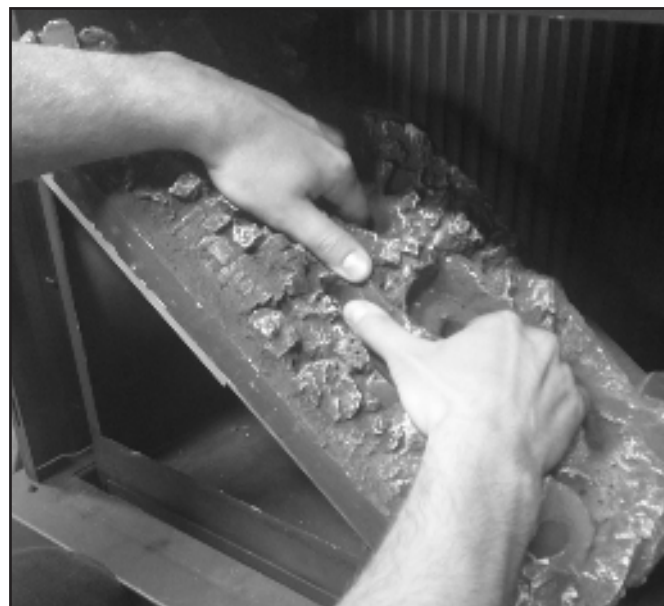
Figure 26. Burner Removal - Rotate 45 degrees
