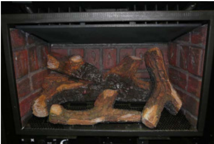
Figure 65. Fourth Stage Log Set Installation.
