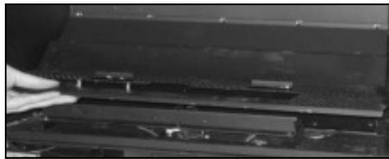
Figure 50: Burner Tray Installation.
