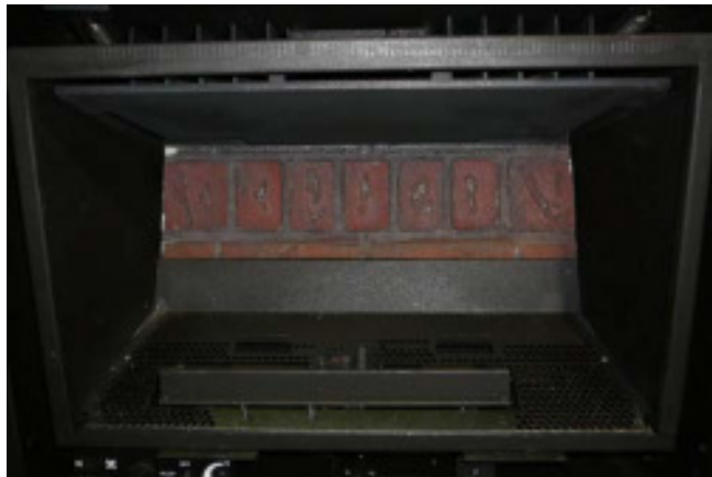
Figure 59: Back Brick Panel in Place.
