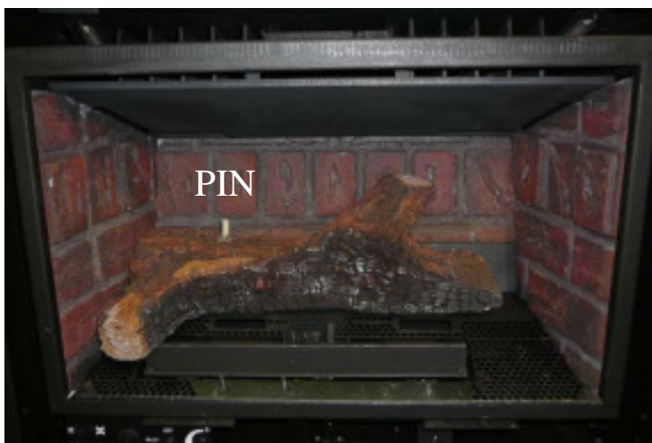
Figure 62. First Stage Log Set Installation.
