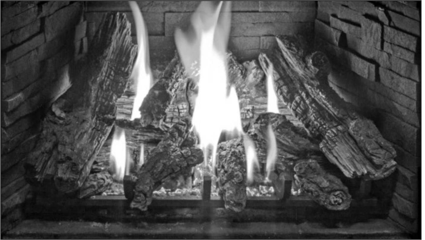
Figure 55: Proper installation and flame appearance
