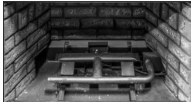
Figure 43: Remove the 6 screws highlighted in figure 42 using a Torx T-20 screwdriver and remove the air deflector
